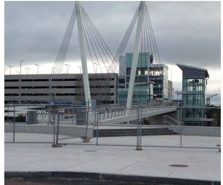
Christina and John Markey memorial pedestrian bridge, Revere
