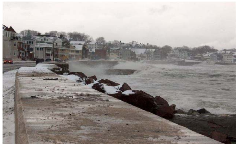
The Winthrop Seawall during a winter storm.
