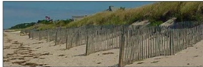
Sand fencing was installed along the base of and perpendicular to this eroded dune to trap windblown sand and help rebuild the dune. [Photo: CZM]
